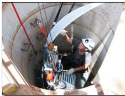
Ribbon profile being fed into the winding unit
