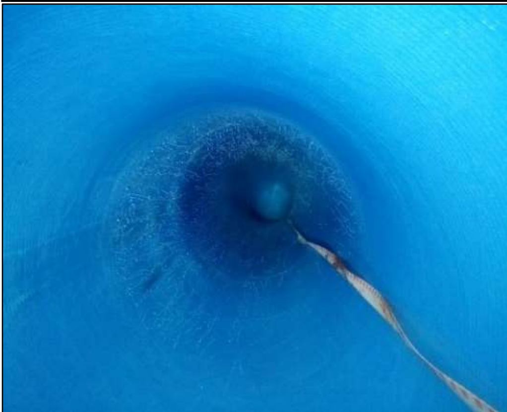
Installed 500NB CIPP Liner
