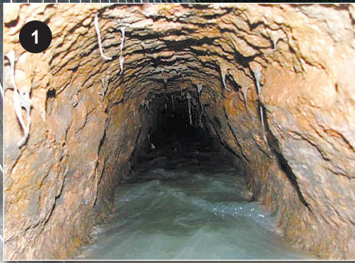
Before (pic 1) and after (pic 2) trenchless pipe replacement.
