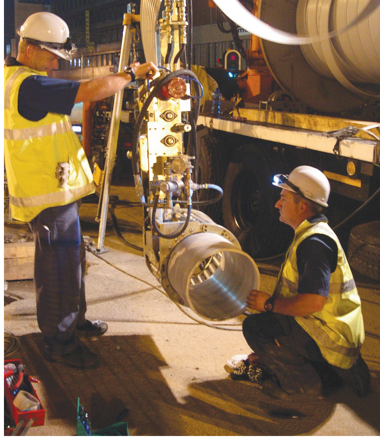
Preparation of Expanda winding cage.
