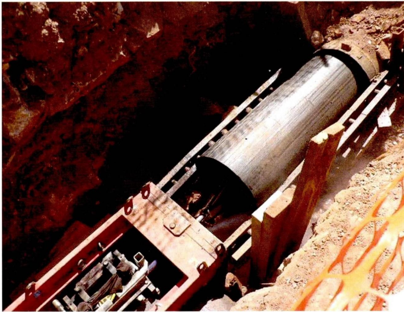
LEFT Completion of sliplining line 1 using 60 t rod puller
